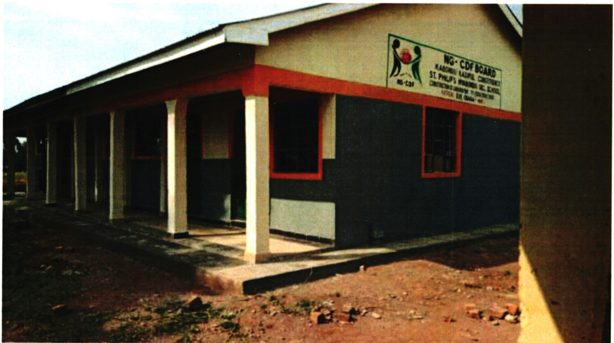
Fig 4: St. Philip's Nyabondo Secondary School: Construction of a Science Laboratory
