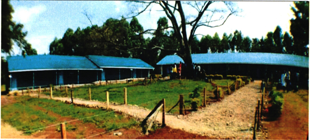
Fig 3: Ringa Primary School: Rehabilitation of 14 Classrooms
