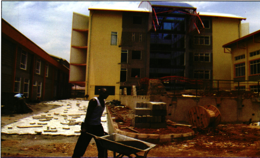
Buru buru library under construction
