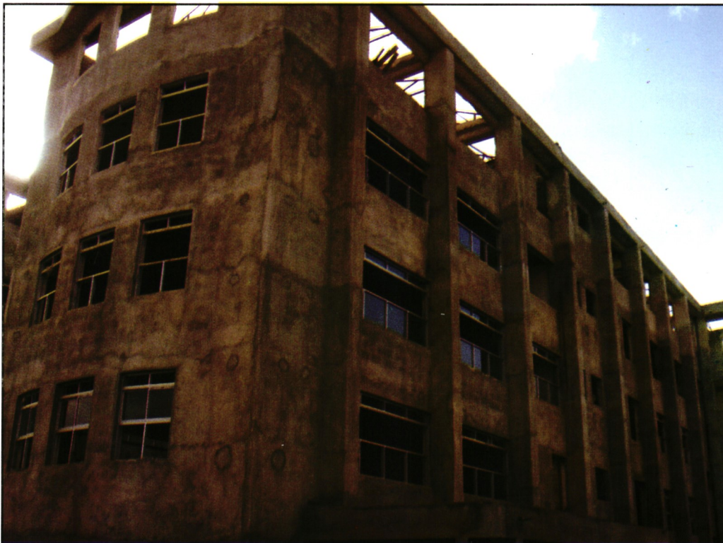
Nakuru library under construction
