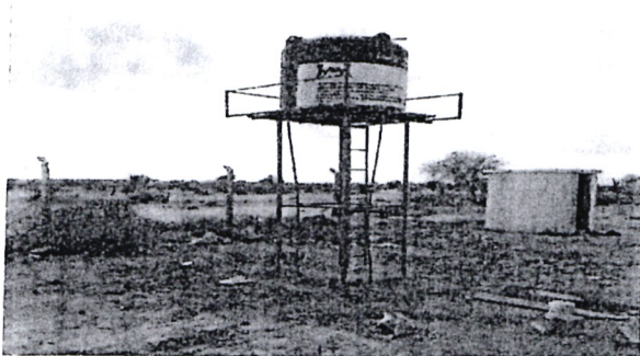
Construction of elevated water tank at Diff Deputy County Commissioner office
