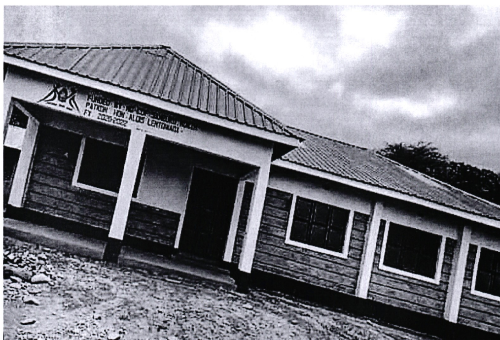
Arsim primary school administration block
