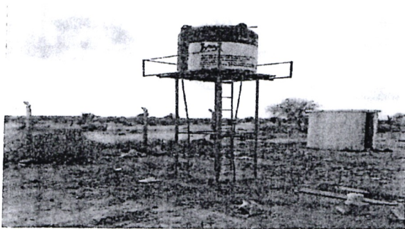
Construction of elevated water tank at Diff Deputy County Commissioner office
