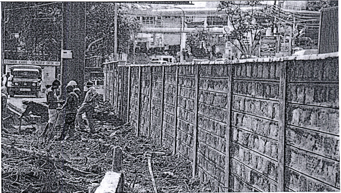
Figure 3: Parklands Police Station- Construction of perimeter wall
