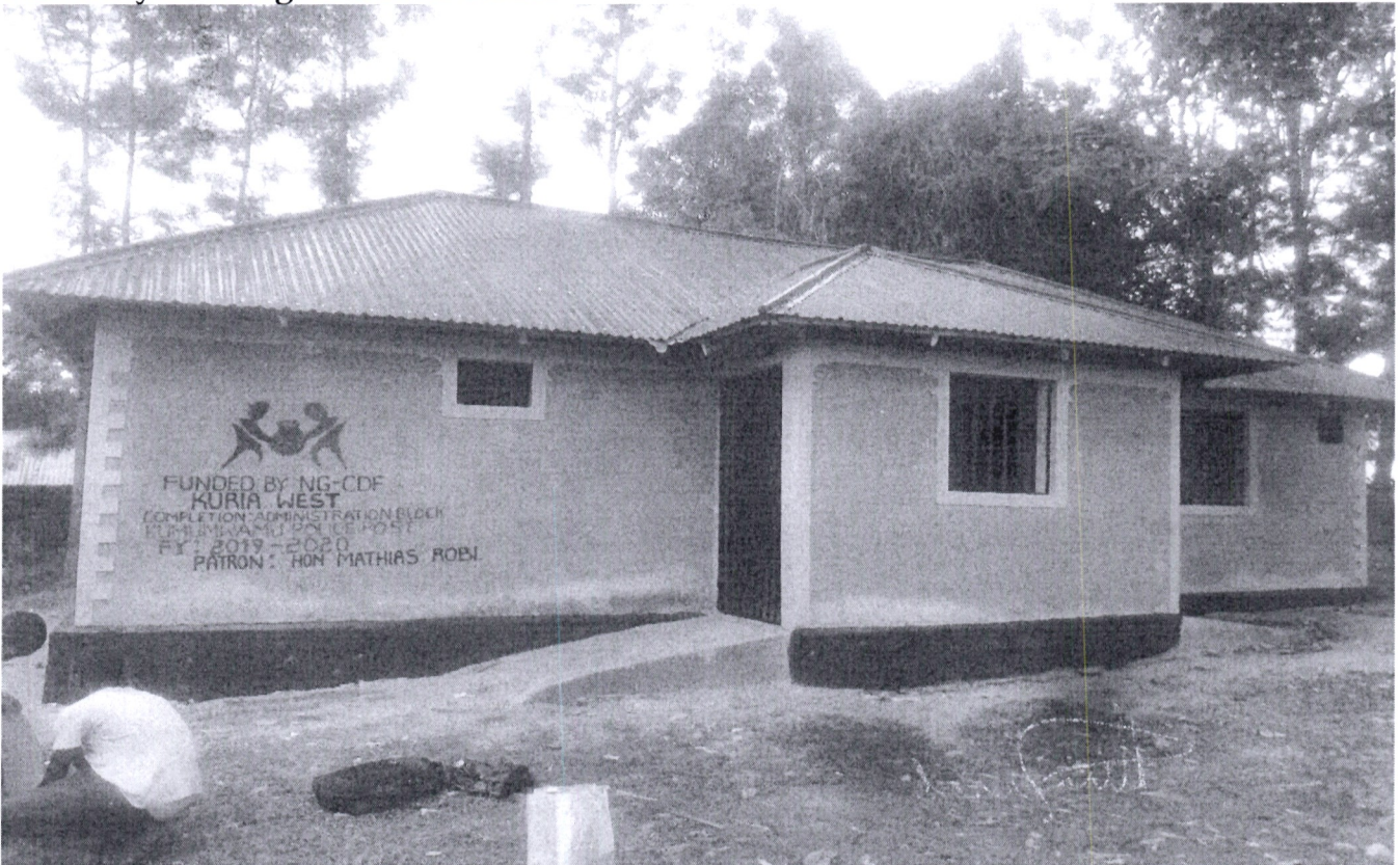
Above: Kumunwamu police line administration block
