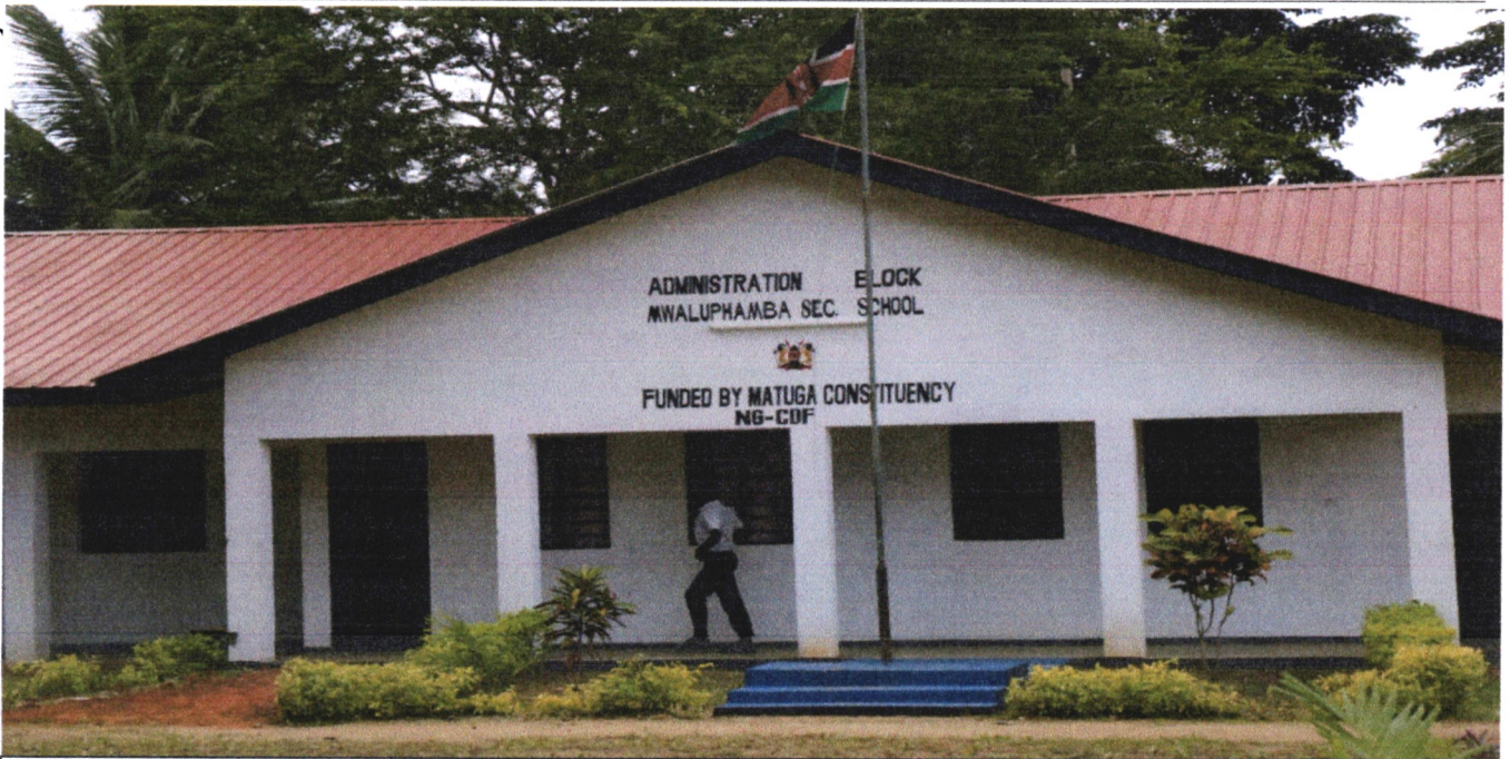
Project name: Mwaluphamba Secondary School Financial Year: 2018/2019 Activity: Completion of Administration block Amount allocated: Ksh 900,000=
