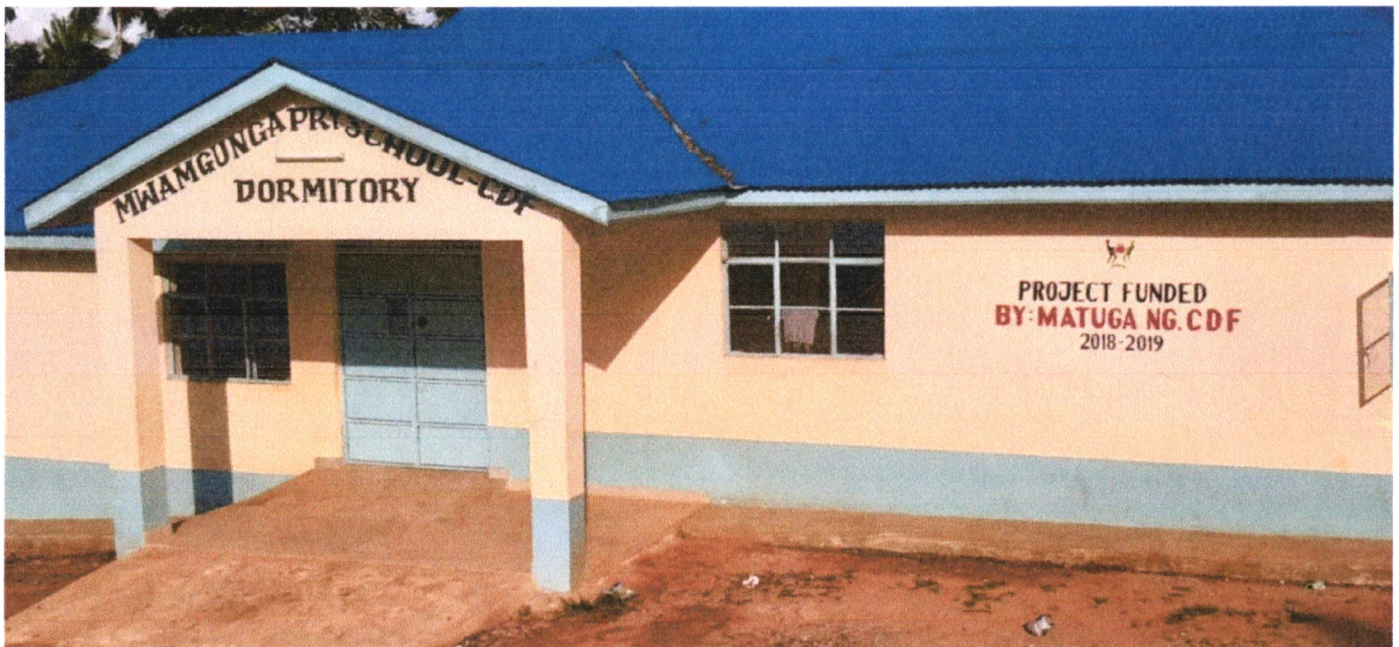
Project name: Mwamunga Primary School Financial Year: 2018/2019 Activity: Construction of a Domitory Amount allocated: Ksh 6,000,000=
