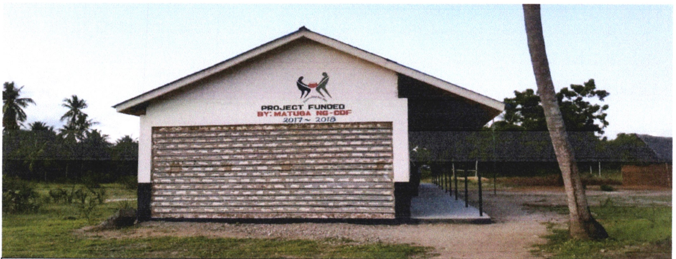
Project name: Madibwani Primary School Financial Year: 2018/2019 Activity: Construction of 3No. Class rooms Amount allocated: Ksh 2,700,000=
