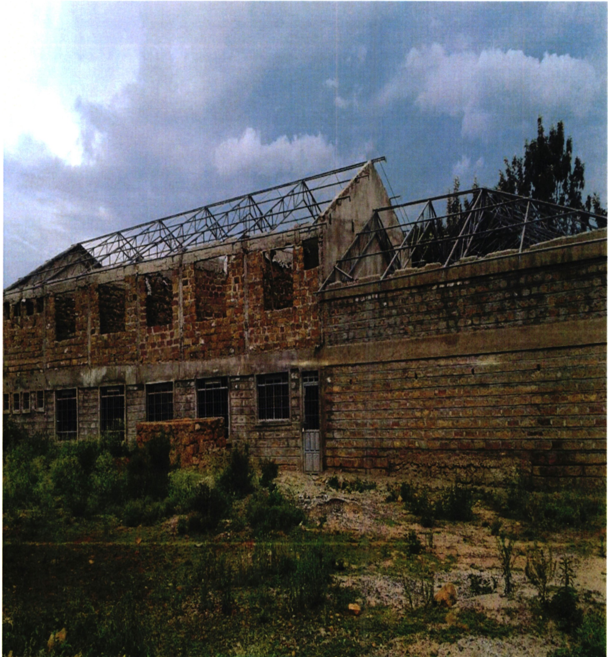
Kabondo Kasipul NGCDF office under construction.
