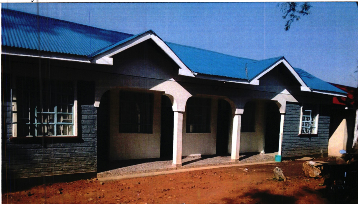
The office is currently house in Kabondo East Chiefs Office
