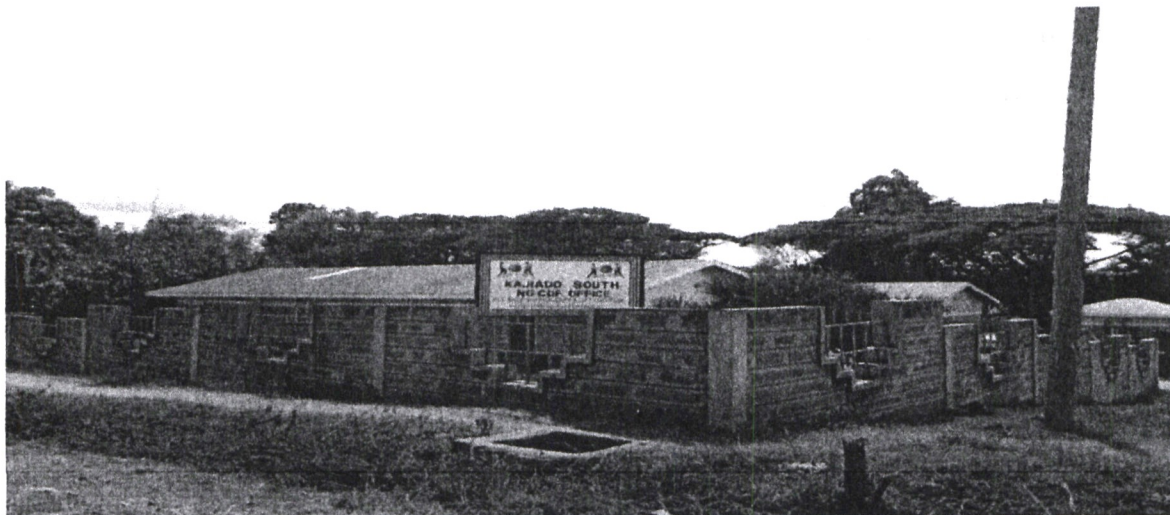
KAJIADO South constituency offices
