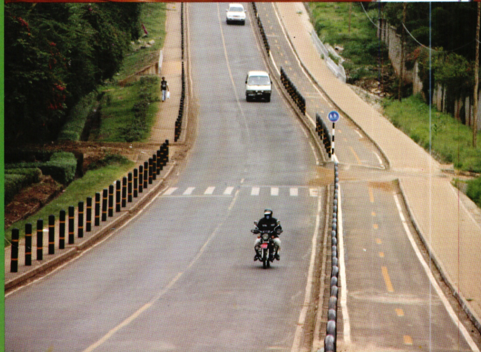
Below: A section of Rehabilitated UN Avenue showing Non-Motorised traffic: cycle lane, footpath and the carriageway
