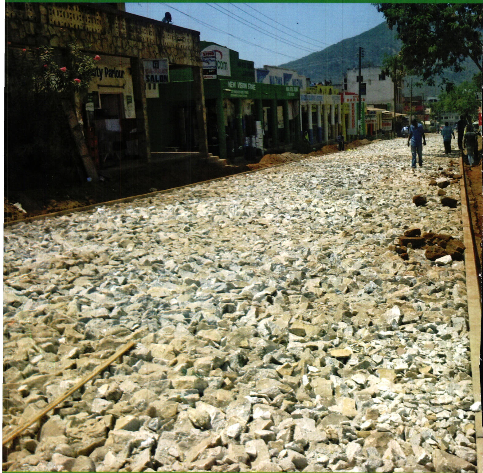
Upgrading of Poster Road in Voi
