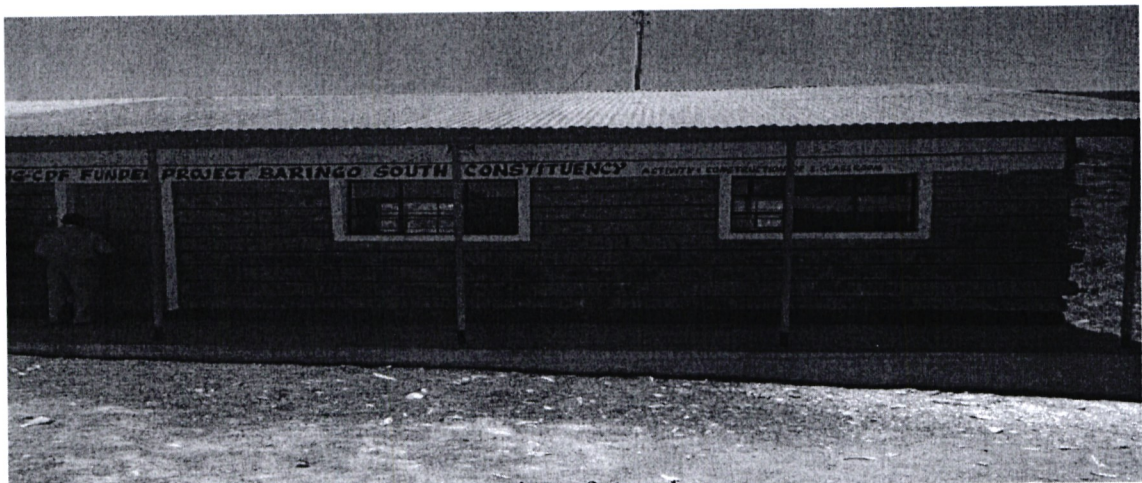
Kimoigut primary school- construction of one classroom
