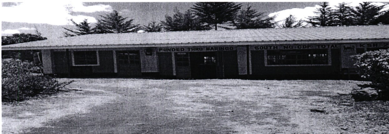
Mwenge secondary school – Construction of laboratory and equipping
