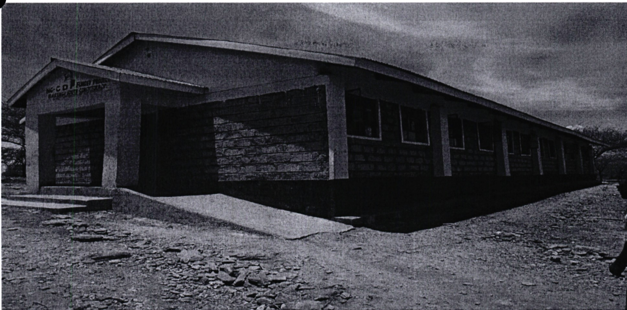
Maoi primary school- construction of boys dormitory
