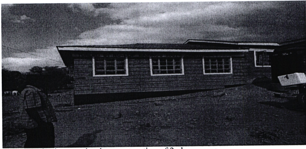
Kamungei primary school – construction of 2 classrooms
