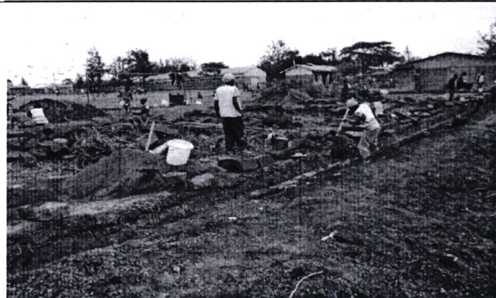
COMPLETION OF PERIMETER WALL ON-GOING AT KIBOWEN KOMEN PRIMARY SCHOOL
