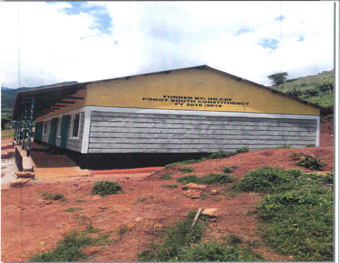
Fig. 1: Kochiy Mixed Day Sec. School, 2 Classrooms
