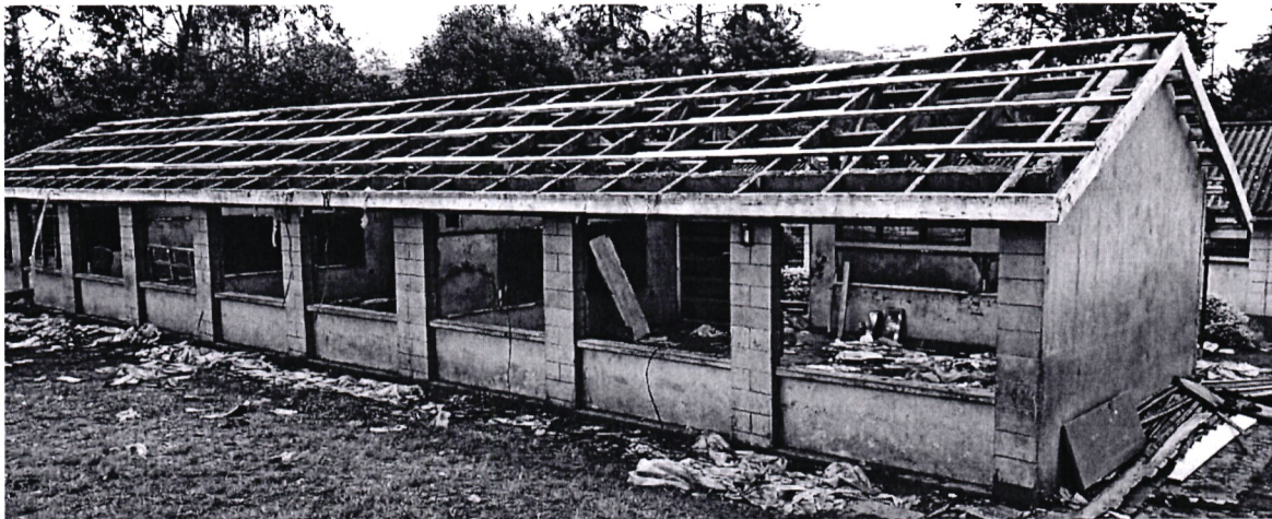
Ngong Forest Primary School – Before renovation
