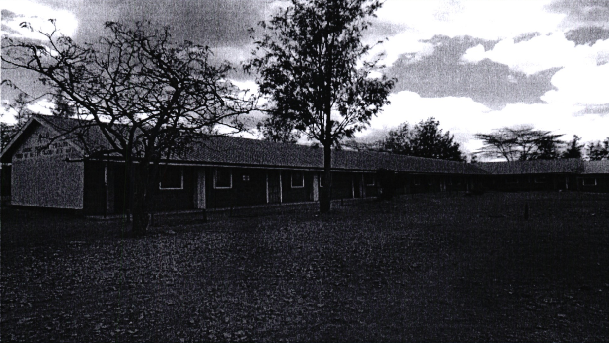
FIG 1.3: RENOVATION OF SIX CLASSROOMS AT NDEMI SECONDARY SCHOOL LEADING TO CONDUCTIVE LEARNING ENVIRONMENT FOR THE PUPILS
