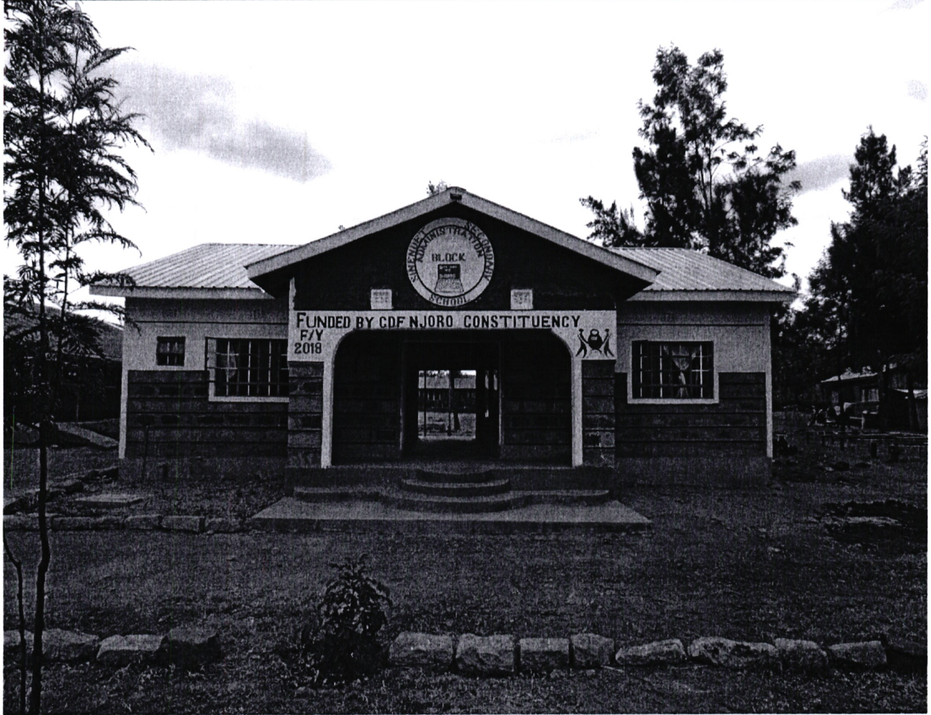
FIG 1.2 CONSTRUCTION OF SINENDET SECONDARY SCHOOL ADMINISTRATION BLOCK FOR SERVICE DELIVERY IMPROVEMENT.
