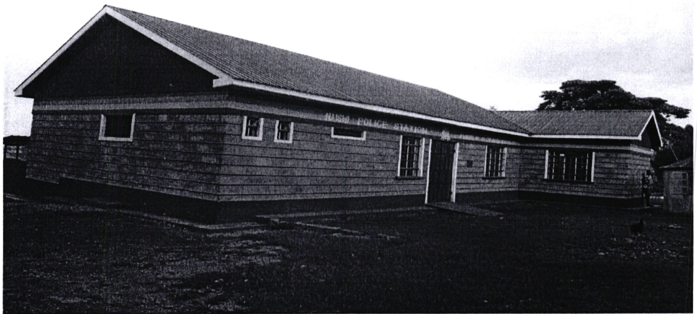
FIG 1.1: CONSTRUCTION OF NAISHI POLICE STATION OFFICES FOR EFFICIENT SERVICE DELIVERY
