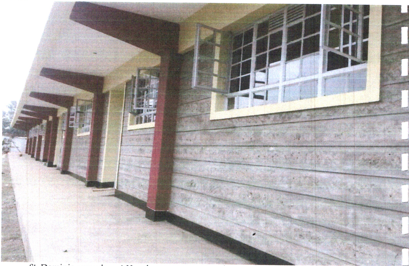
St. Dominic secondary 4 No. classrooms construction
