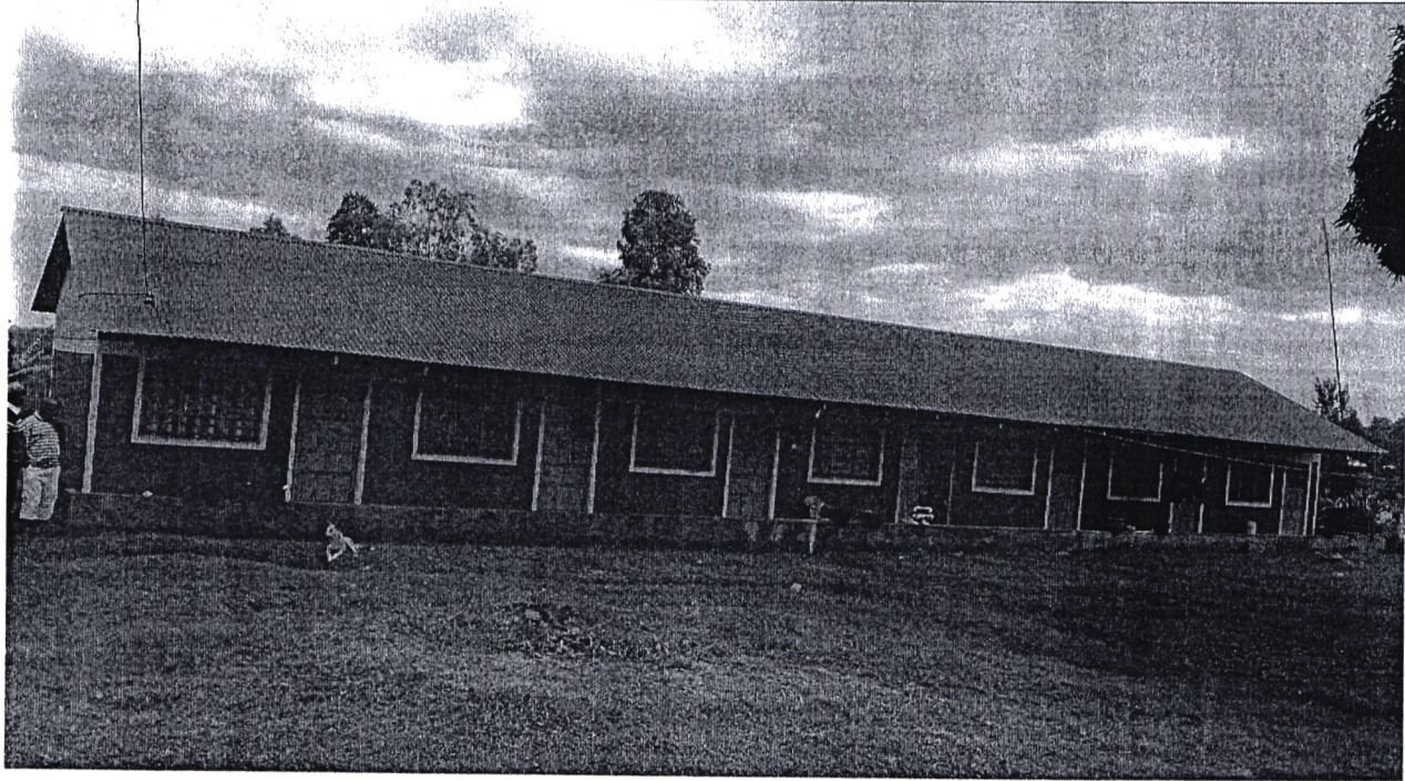
KITUTU CHACHE SOUTH NG CDF PROJECT-7 UNITS OF STAFF HOUSES CONSTRUCTED BY NG-CDF AT RUGA AP. LINE
