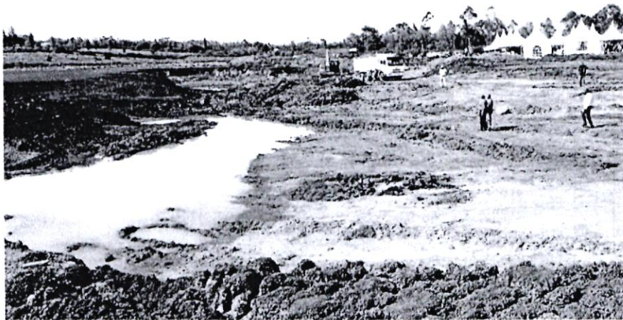
Ongoing construction works on Lusoi dam
