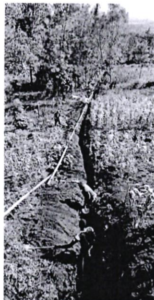
Construction of Simbara-Kamatongu Pipeline
