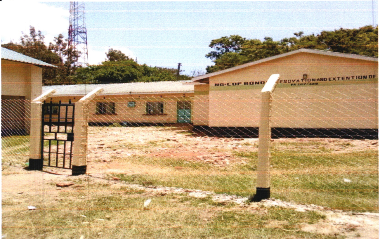
BONDO NGCDF OFFICE RENOVATION
