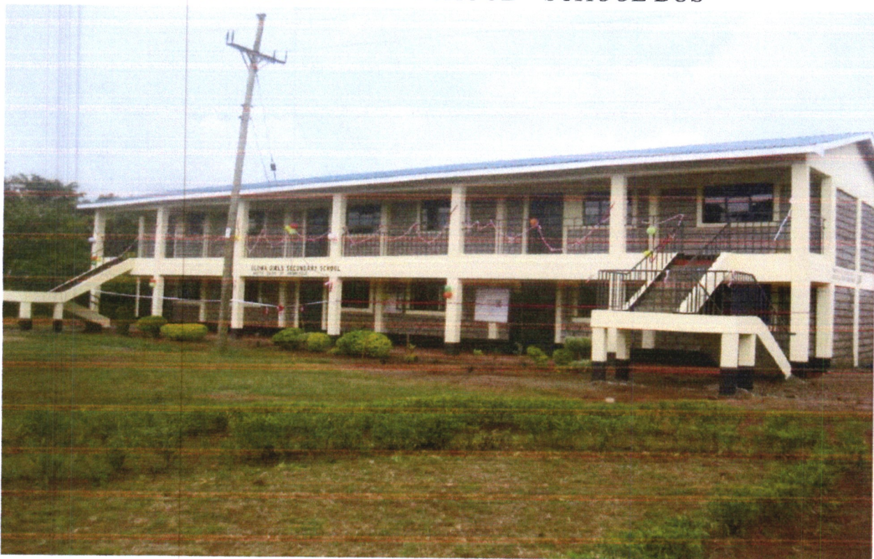
ULOWA GIRLS SECONDARY SCHOOL (CONSTRUCTION OF 6 CLASSROOMS)
