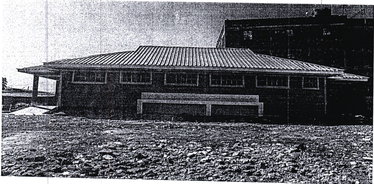
Kibera Primary School Ablution Block
