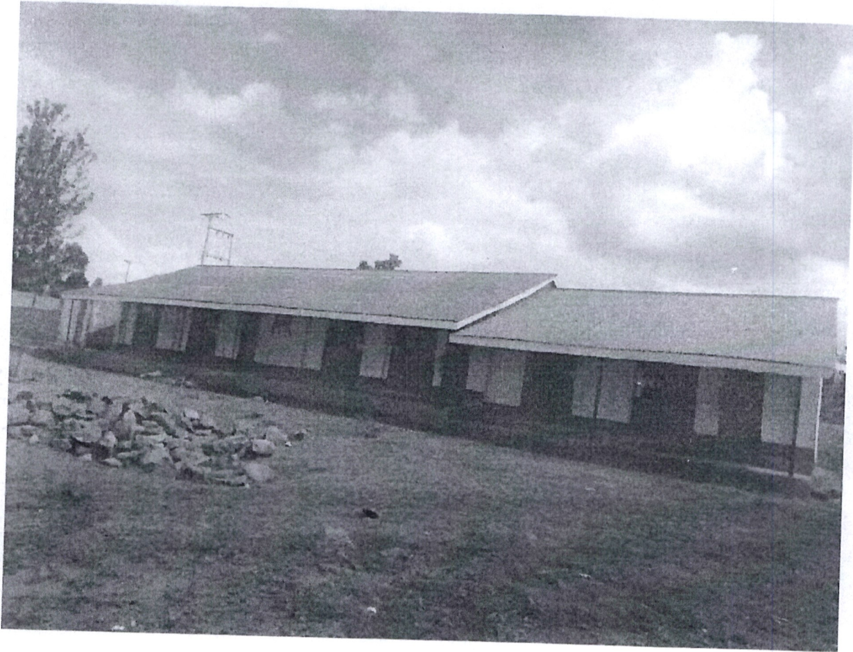
Figure 4: Andingo kodit two classrooms complete in FY 201819
