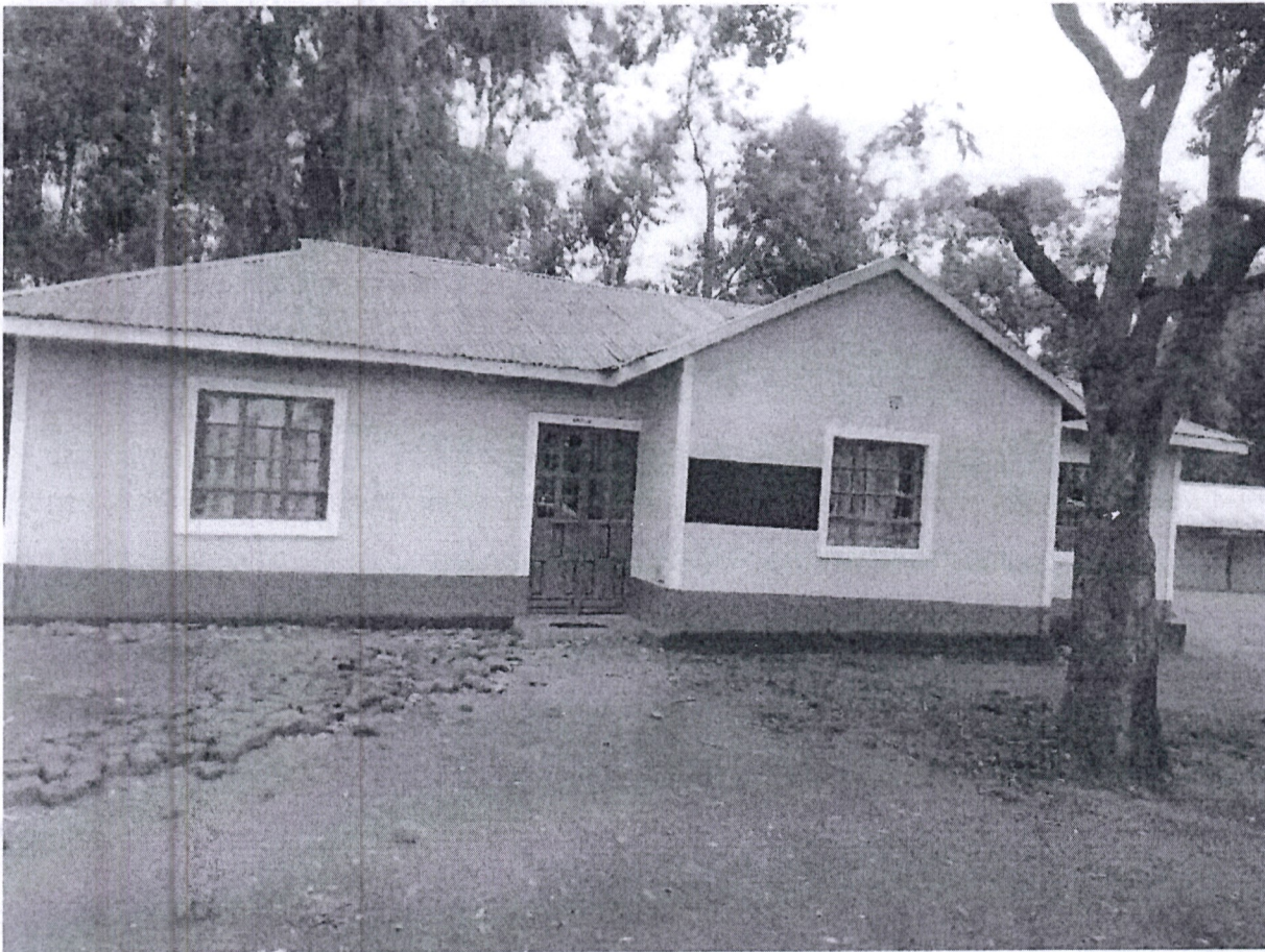
Figure 3. Radienya Primary school Administration Block completed in FY 2018/19
