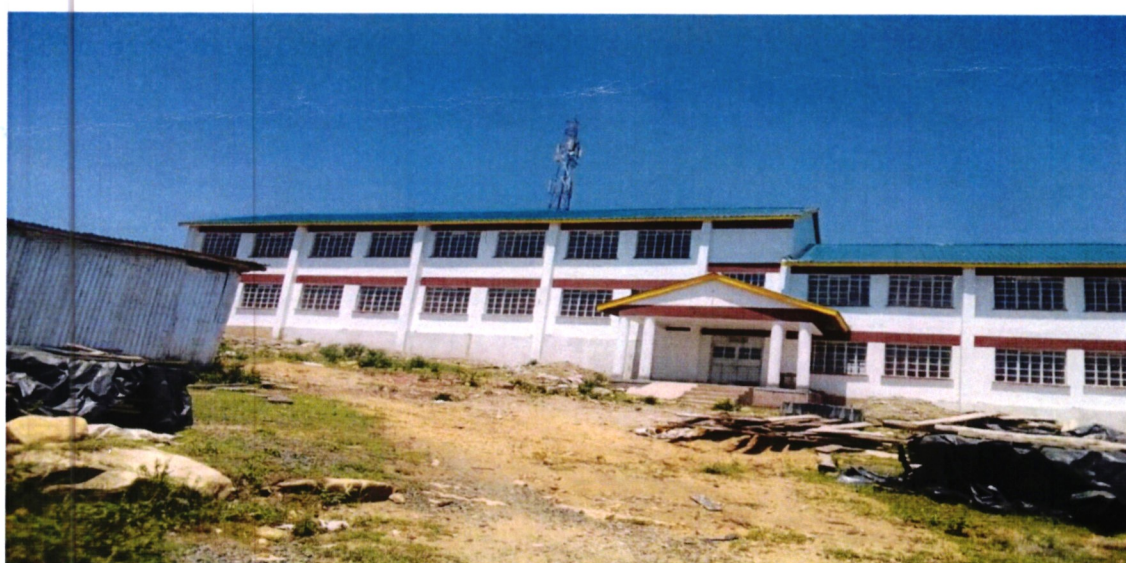
KMTC Navakholo – construction of administration block
