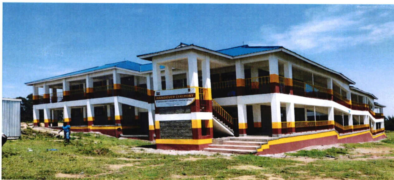
KMTCC Navakholo – Construction of Storey building of 12 lecture halls in Bunyala Central Ward, complete and handed over
