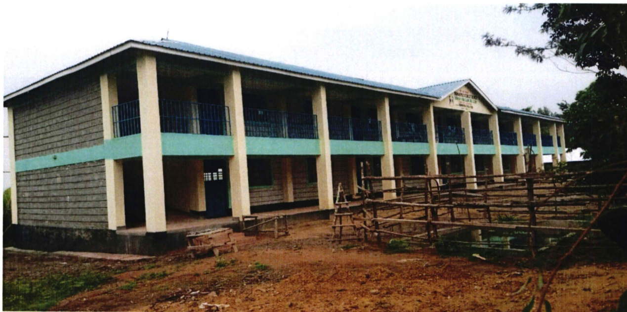
Buhayi Muslim Secondary School – construction of one storey building of 8no. classrooms in Bunyala West Ward, complete and handed over but final payment will be done in 2021/2022 FY
