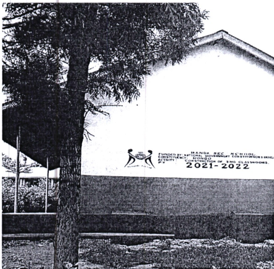
BANDA MIXED SEC SCHOOL CONSTRUCTION OF 3No. CLASSROOMS
