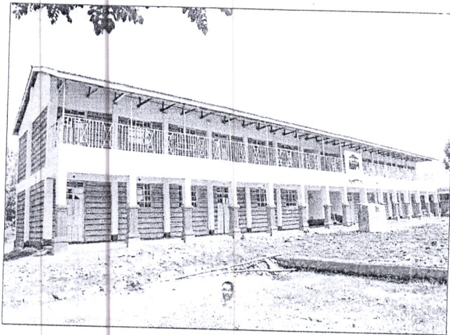
Matili Primary Schools (8 Classrooms Storey Classrooms)
