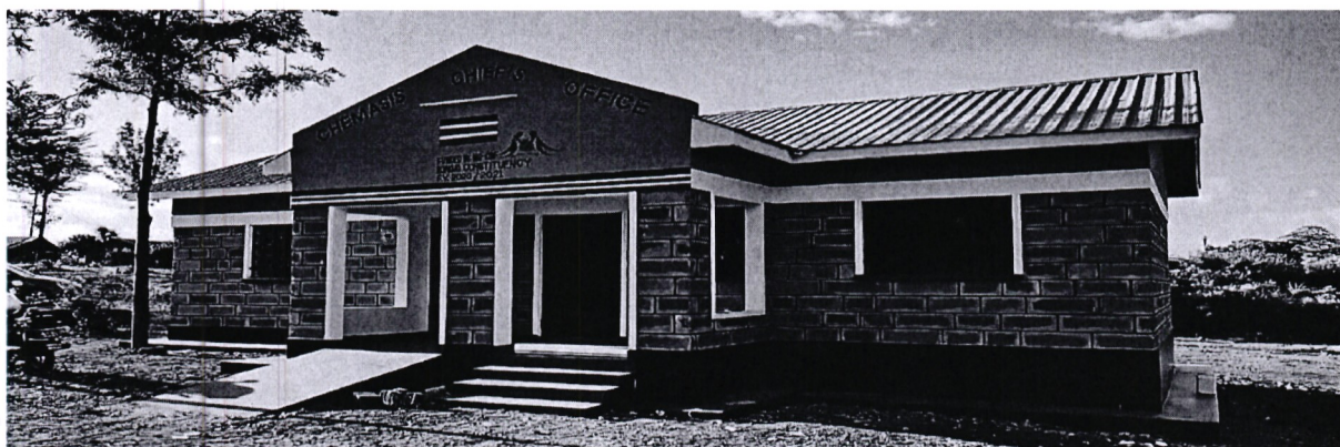
Image 1: Chemasis Chief's Office; Construction of a chief's office to completion.
