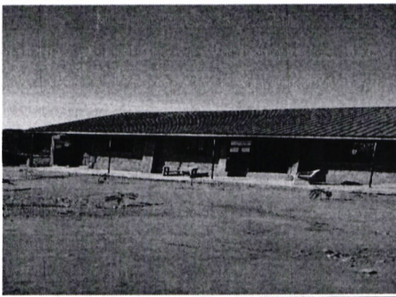
FIG 1.1: One Classroom constructed at Makutano Secondary School FY 2017/2018, to improve learning.
