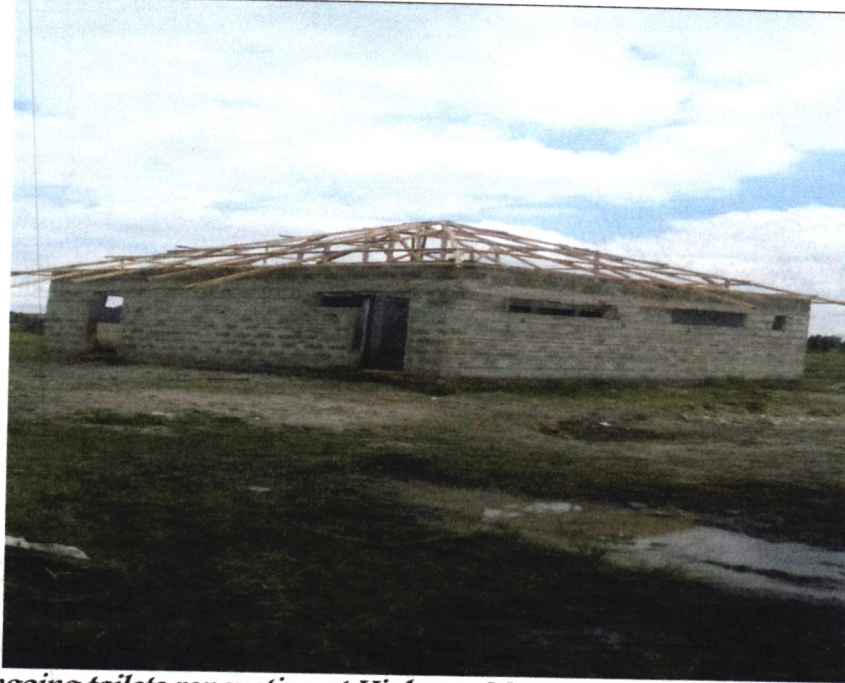
Ongoing toilets renovation at Highway Manyatta Primary School
