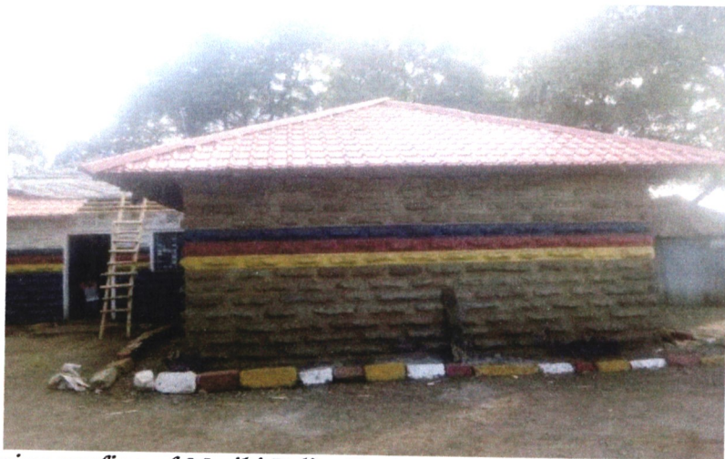
Ongoing roofing of Mwiki Police Post
