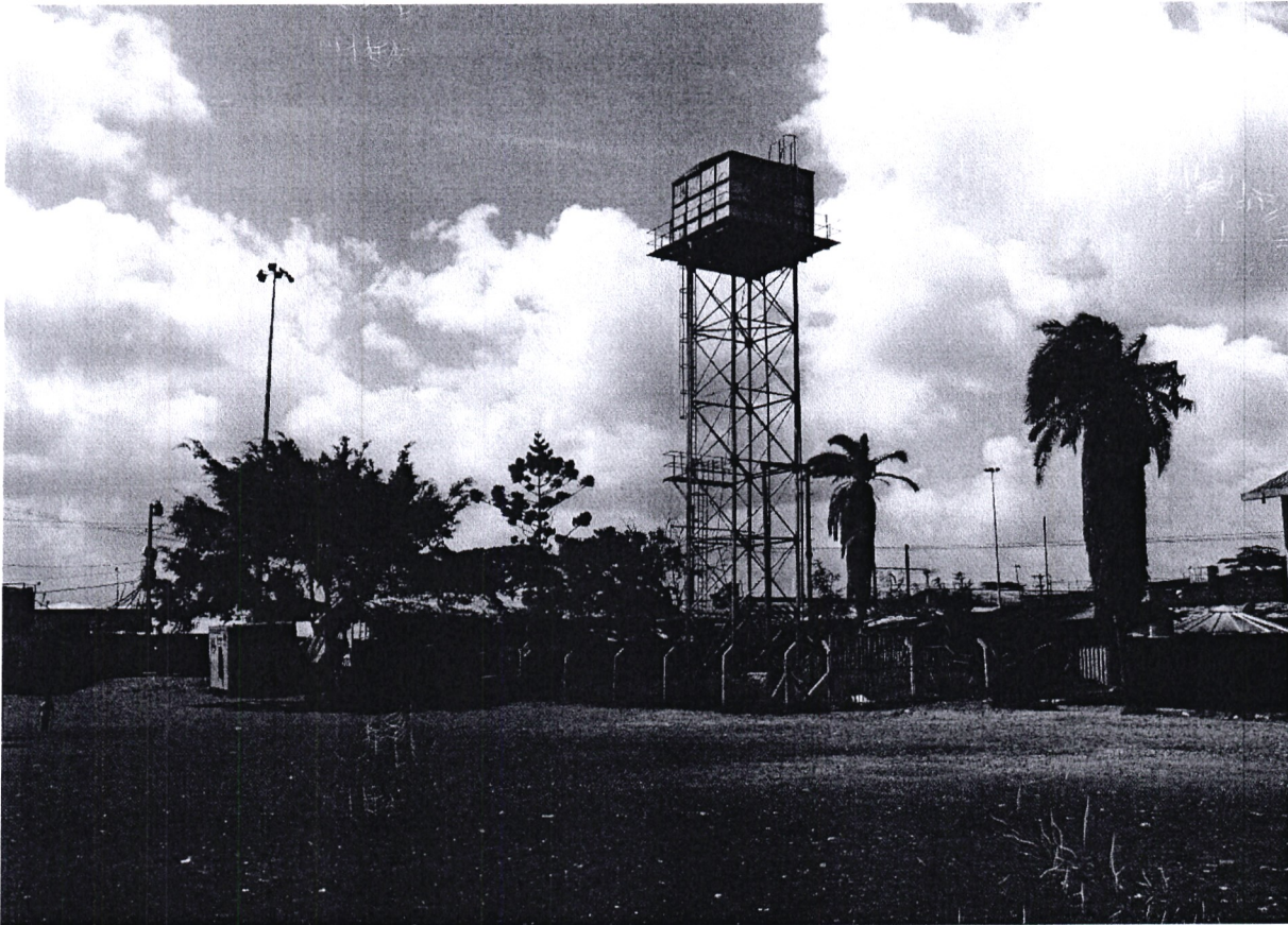
Star of Hope Secondary school borehole
