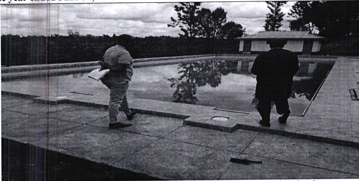
Construction of a Swimming Pool at Gatanga Girls High School
