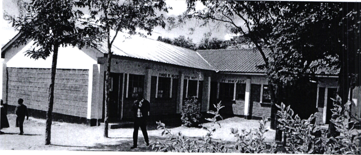
Construction of 3 classrooms in Kitamwiki Primary School
