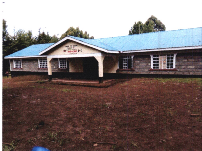
TABAIN PRIMARY SCHOOL-CONSTRUCTION OF ADMINISTRATION OFFICES AND 2 CLASSROOMS-KAMARA WARD
