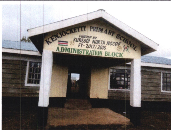
KENJOCKETTY PRIMARY SCHOOL-CONSTRUCTION OF ADMINISTRATION OFFICES AND 2 CLASSROOMS-NYOTA WARD
