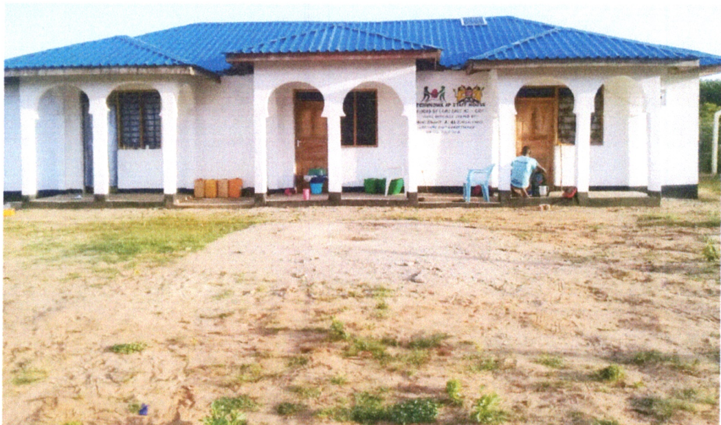
2. Tchundwa AP houses being the first permanent humane accommodation for the police; 6 roomed house with chain-link fence and two blocks of toilets
