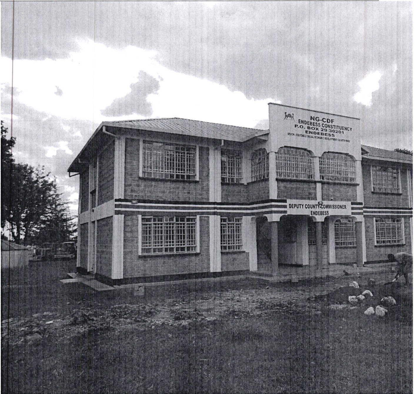
A Front View of newly constructed NG-CDF offices at Endebess town.
