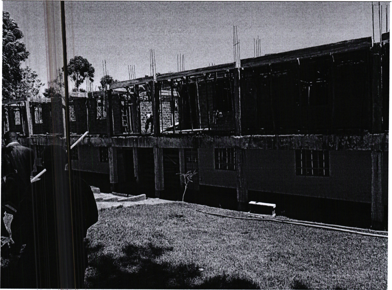
Riokindo Primary School at cost of 19m and will be completed by Decemeber,2018
