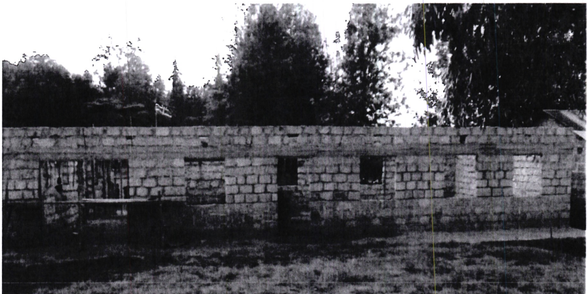
Ongoing Kiptuno Primary School administration block
