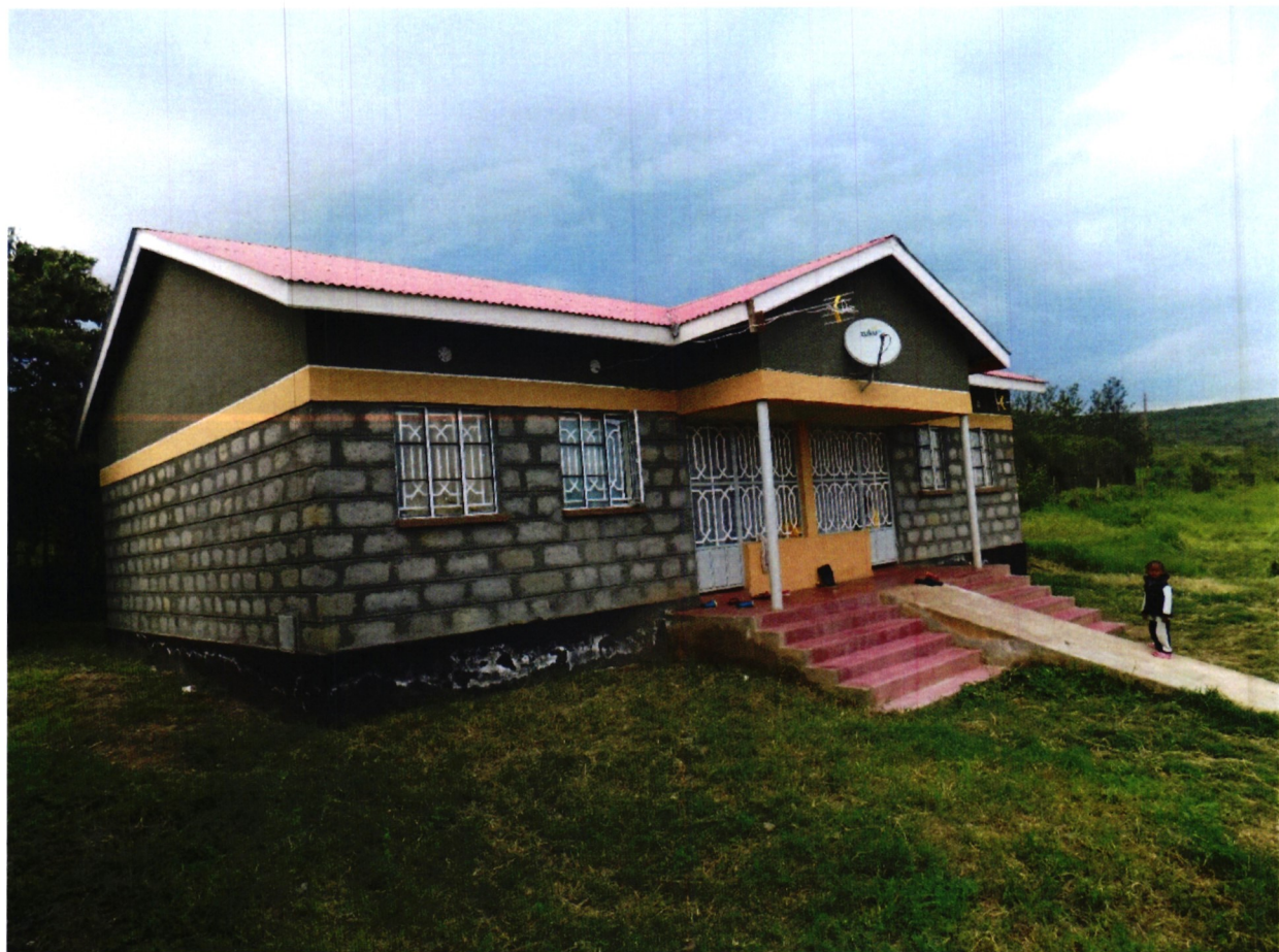
Fig: 3-Kikopey Secondary school one-bedroomed complete and in use (Staff house)
