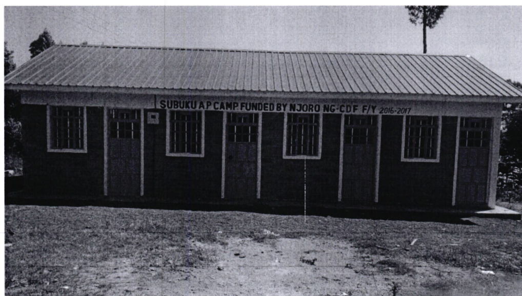
FIG 1.3: Construction of an AP camp at Subuku Location in Kihingo Ward.
