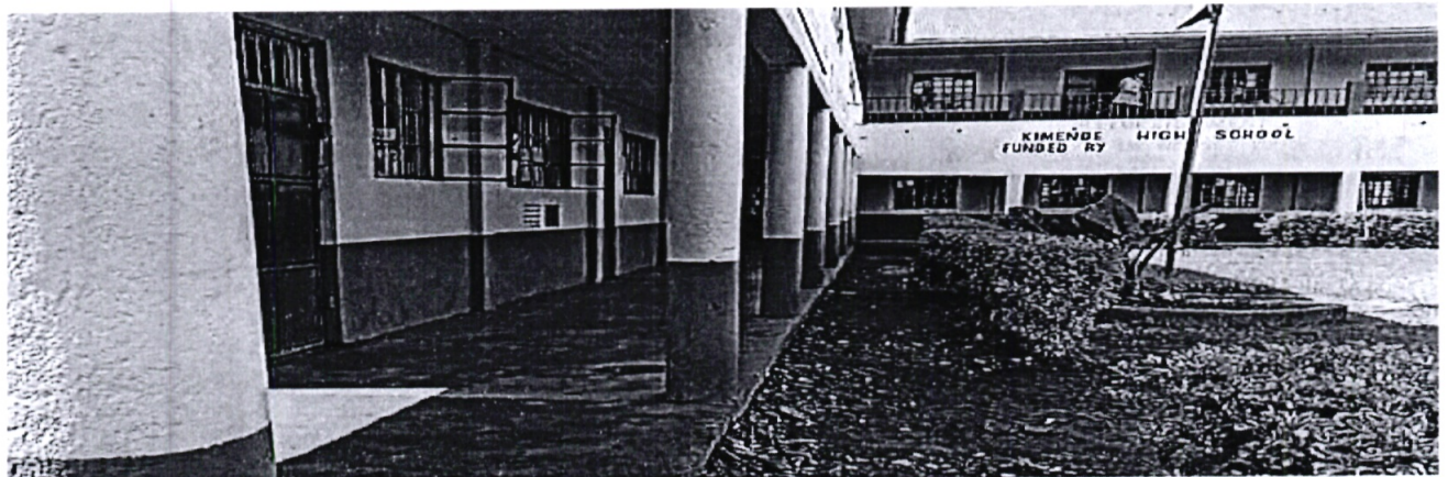
Kimende high school Renovation of the whole school
