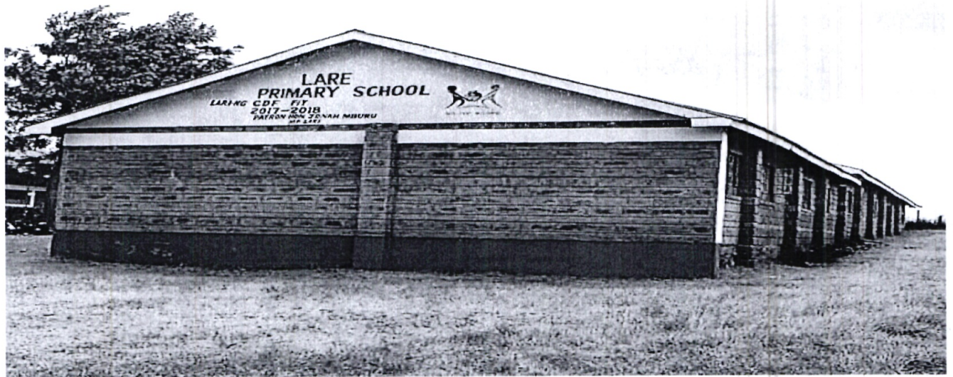
Lare primary school Renovation and construction of the school
