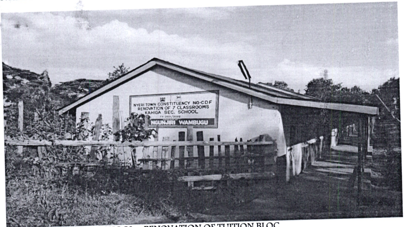
KAHIGA SECONDARY SCHOOL – RENOVATION OF TUITION BLOC
