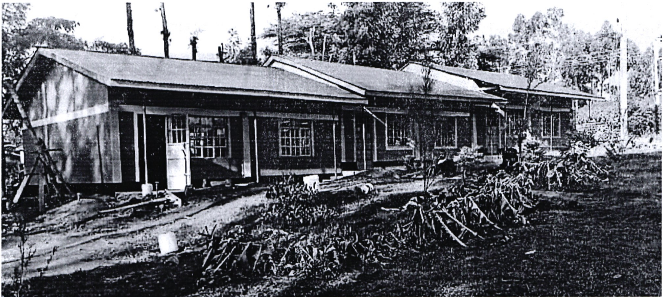
KITUTU CHACHE NORTH NG CDF PROJECT-3 CLASSROOMS CONSTRUCTED BY NG-CDF
