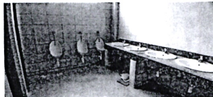
A section of the washrooms in the new Administration block
