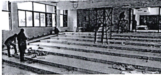
Finishing touches on the new Administration block
