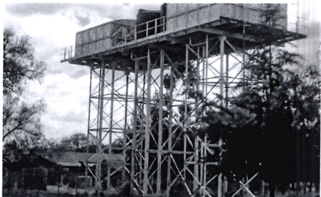
Water reticulation at Lanet in Nakuru
