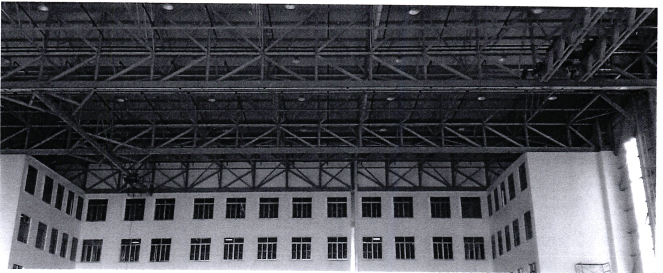
Exterior and interior view of the VVIP Hangar at Embakasi
