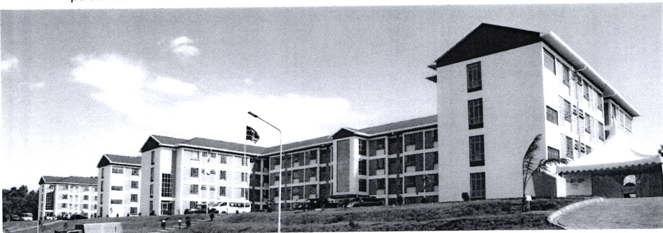
Warrant Officers and Sergeant's accommodation block at Moi Air Base
