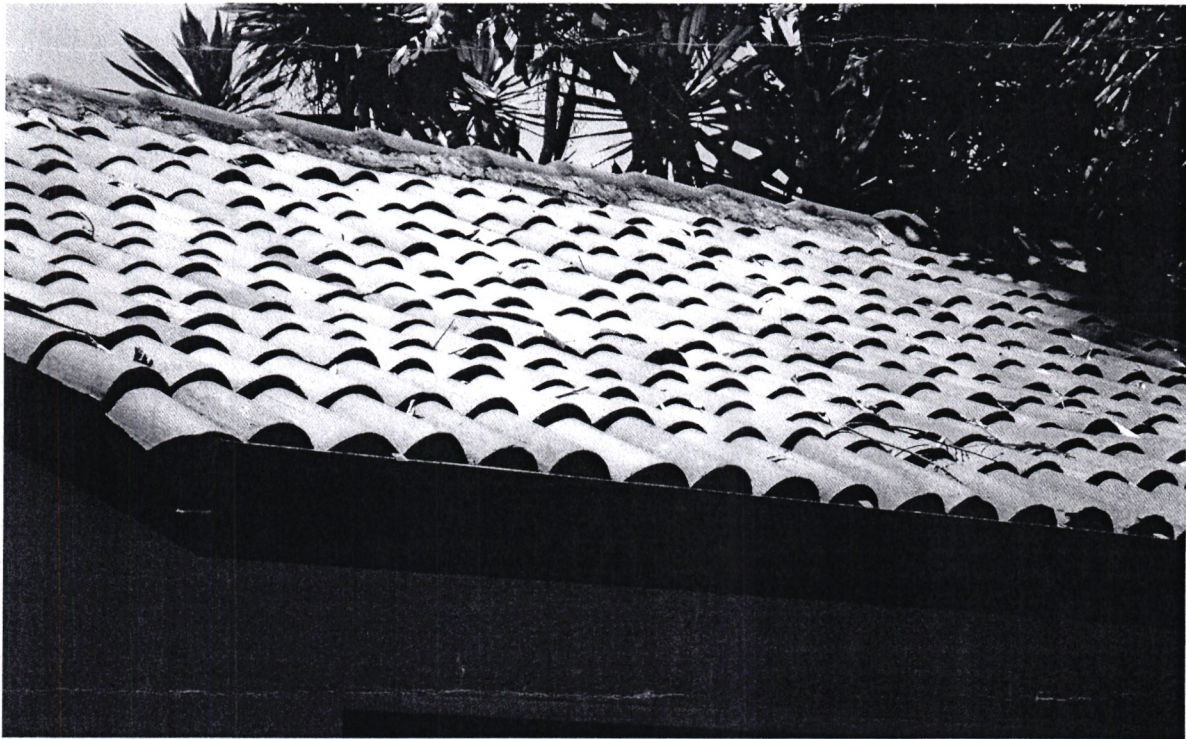
Showing part of the roof
