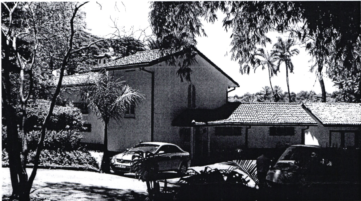
Front view of the property showing the main building
