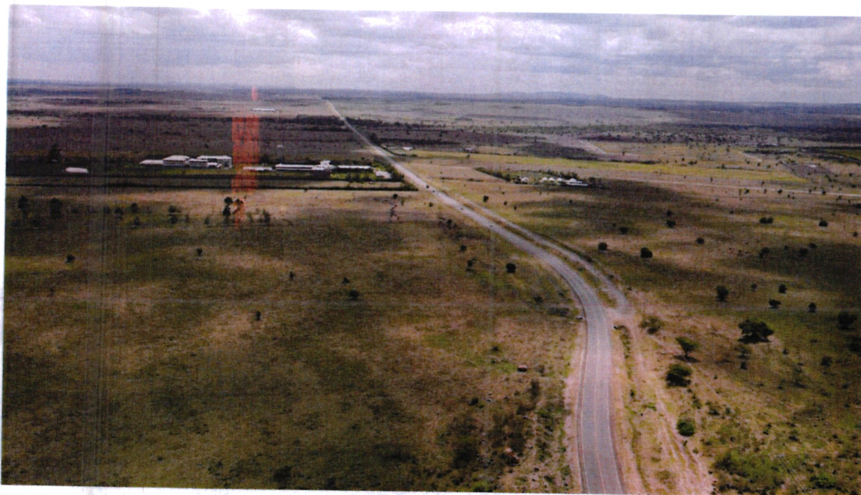
Aerial view of Kiserian-Isinya Road Section
