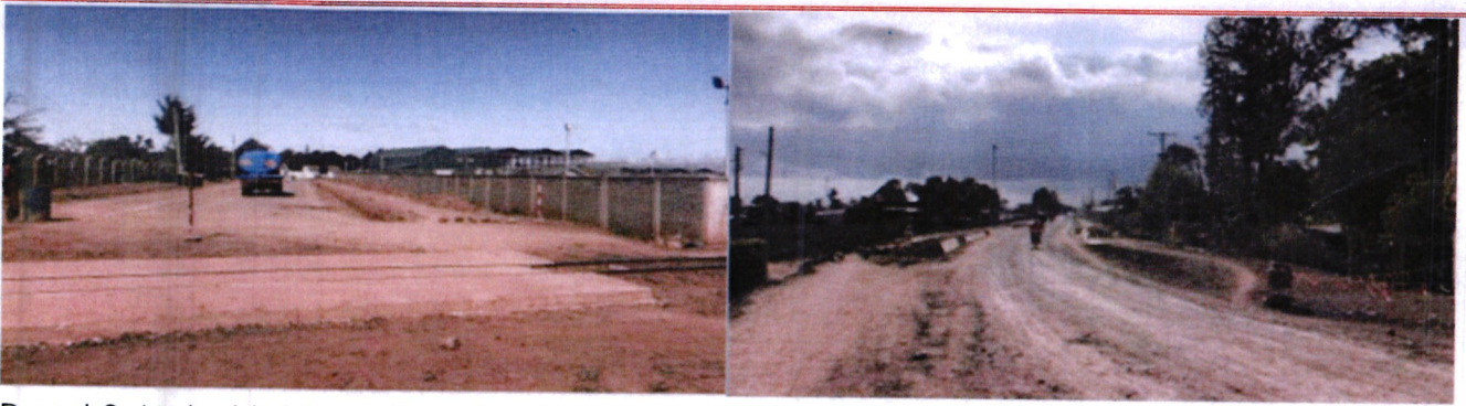
Road 3: Industrial Area Road
