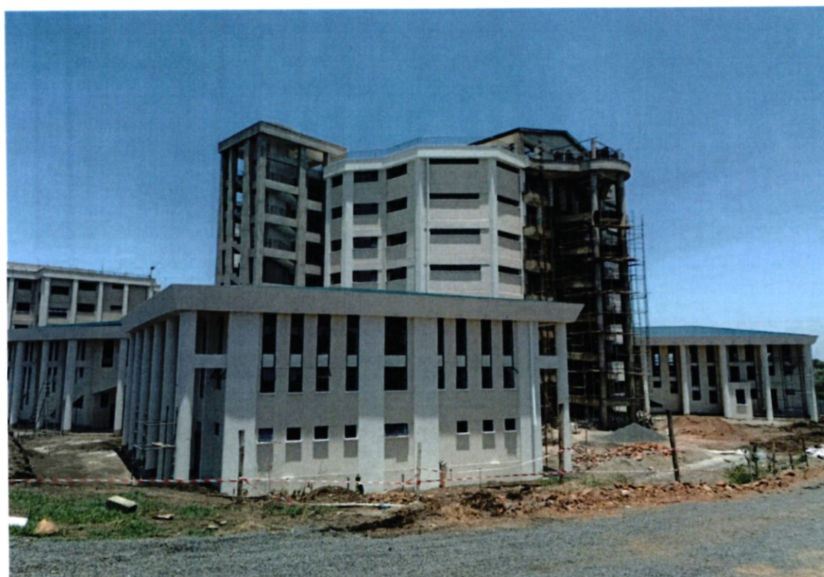
Ongoing Phased Construction of Administration and Lecture Theatres Block
