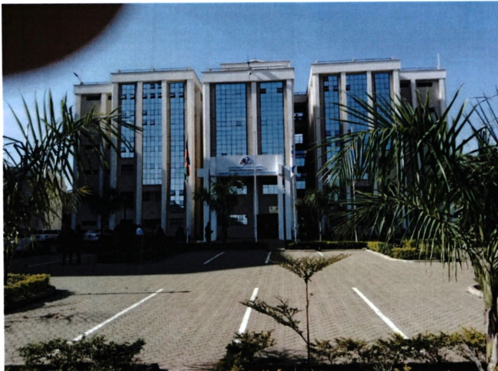
Administration and Lecture Halls Block
