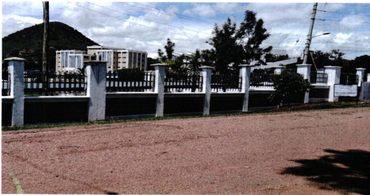
Section of University Perimeter Wall
