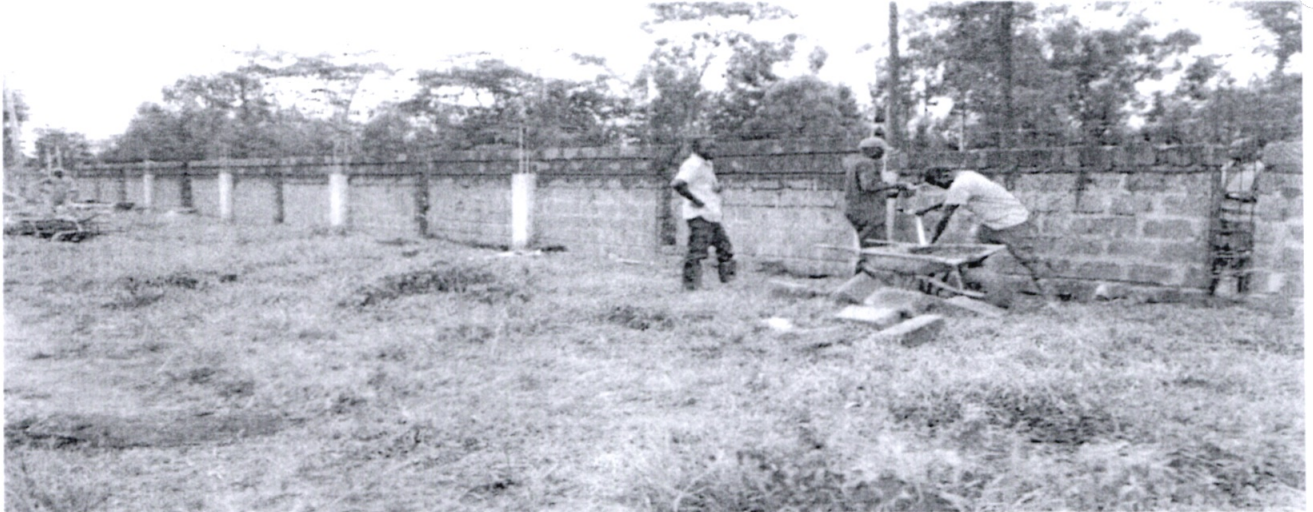
Figure 9: Construction of the College Perimeter wall to enhance security and safety of its property at Ksh 250M.
