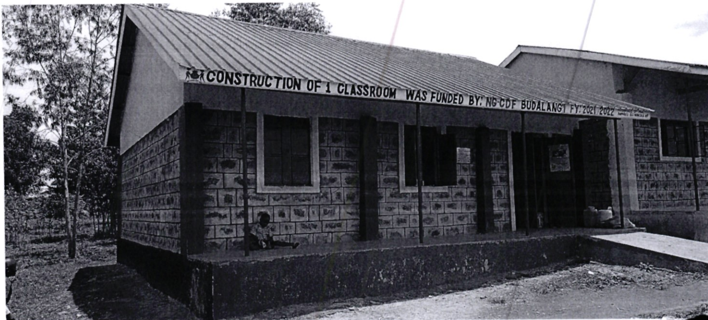
Completed One (1No) classroom at Munani Primary School
