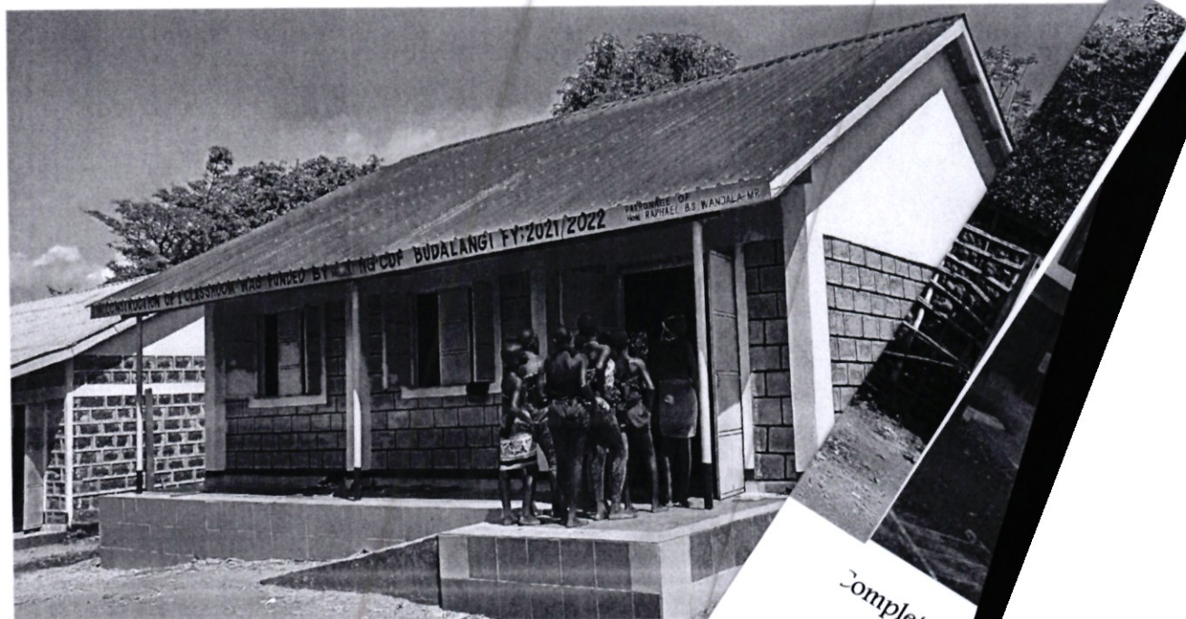
Completed One (1No) classroom at St. Cecilia Primary
