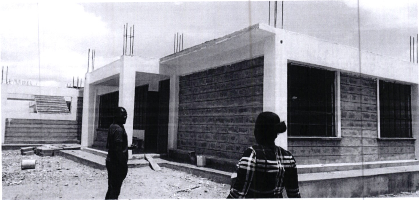
On-going three (3no) storey building at ACK Musoma Secondary School
