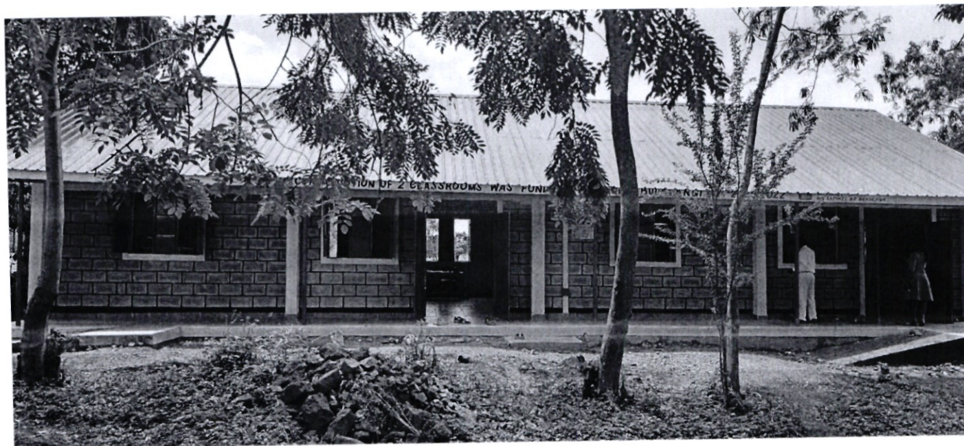
Completed two (2No) classrooms at Bulagu Primary School
