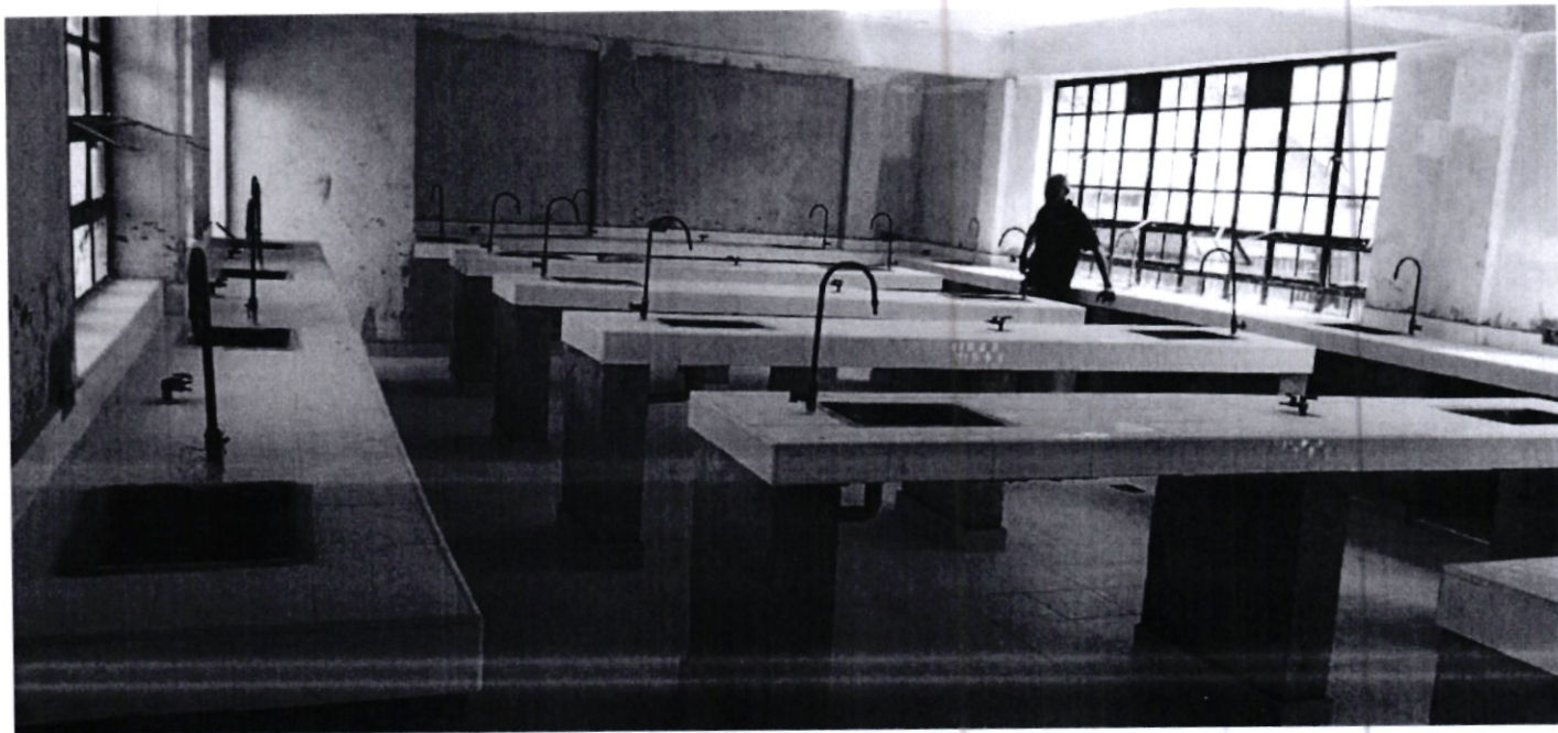
ACK Musoma Laboratory in the On-going 3NO. Storey Building
