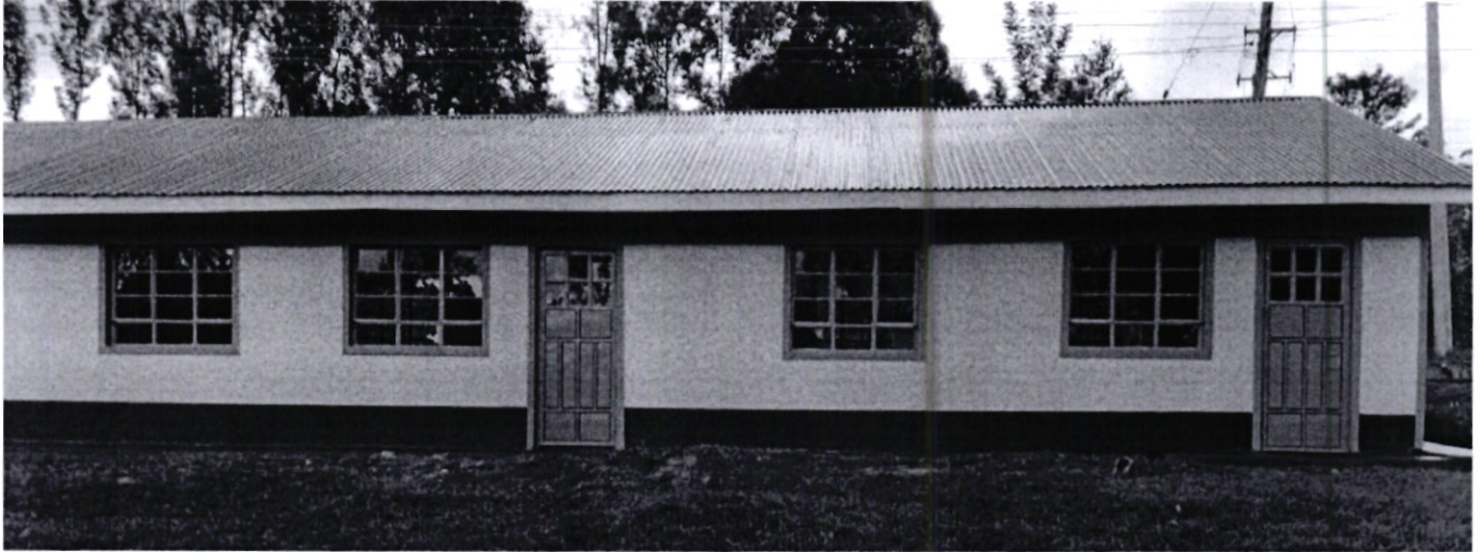
KITUTU CHACHE SOUTH NG CDF PROJECT-3 CLASSROOMS CONSTRUCTED BY NG-CDF AT NYACHOGOCHI PRIMARY SCHOOL
