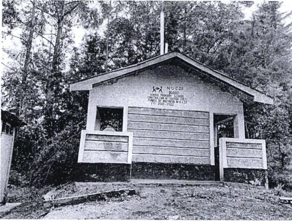
KIRIKI PRIMARY SCHOOL STAFF TOILET BLOCK
